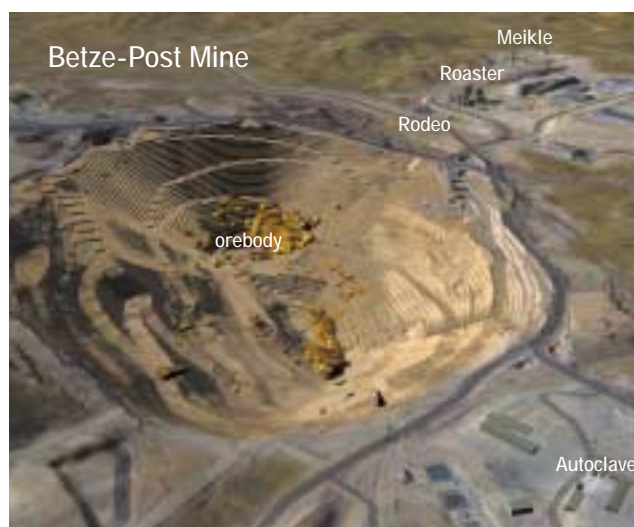
The Betze-Post Mine, a conventional open pit operation located in the southern portion of the Goldstrike Property, is expected to produce 1.61 million ounces of gold in 2001.
