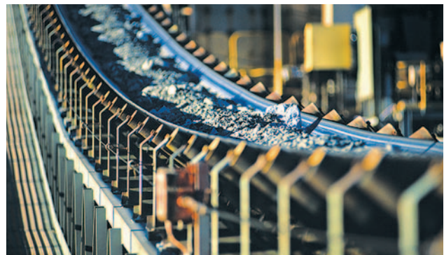
A view of the ore conveyor at the Kanowna asset, which is located close to the joint-venture Kalgoorlie Mine in Western Australia.
