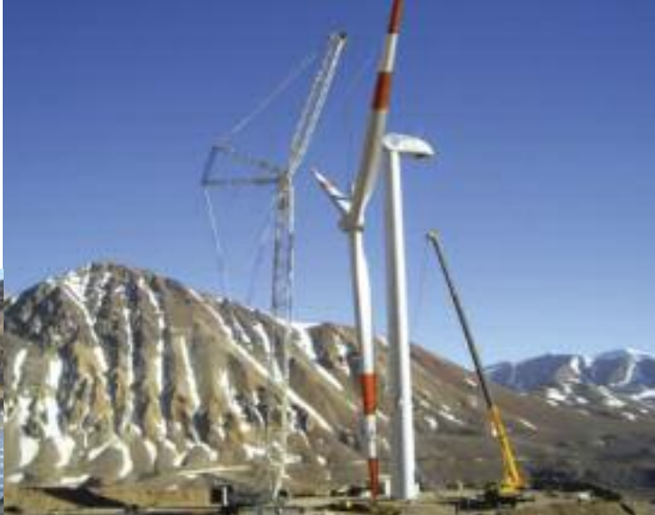
A new two-megawatt wind turbine at the Veladero mine in Argentina will provide renewable energy to the site, testing the potential for wind generation at high altitude. Opposite: Barrick's solar farm in Nevada.
